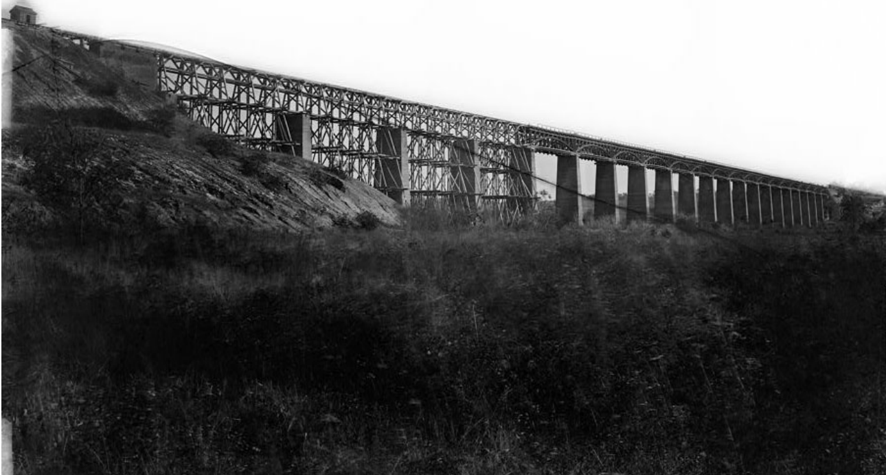
Unique railroad bridge at Farmville, VA The structure on the left end is repair work. The bridge was later replaced with a steel one along side this one. The wood structure of this bridge is gone but the piers still stand. The railroad abandoned the line so the steel bridge is a dramatic part of a rail-trail. The Form19 hopes to do a short article on this bridge & why it had to be repaired.
