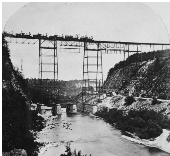
Six engines crossing bridge July 31, 1875. The structure below the top level and to the right were bracing used during construction and would later be removed.
