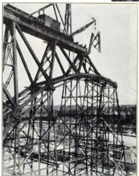
FIG. 3.—ERECTION OF WEST ARCH, ST. CROIX RIVER BRIDGE.
