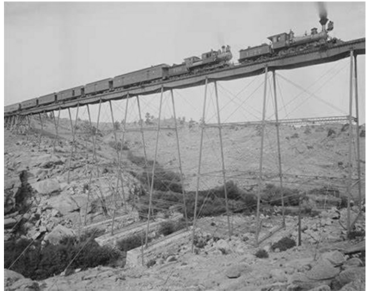
Dale Creek Bridge in SE Wyoming -original above replacement on the right. Both steadied by cables
